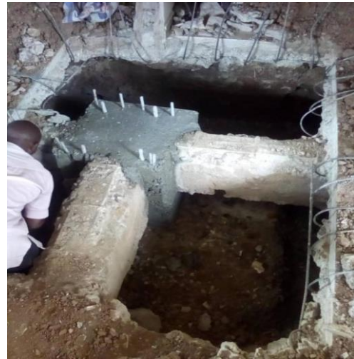
Ongoing work on the tower
